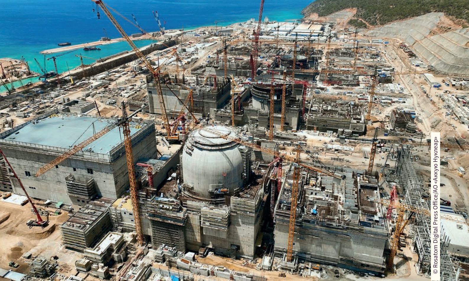
Construction of Akkuyu nuclear power plant in Turkey.
