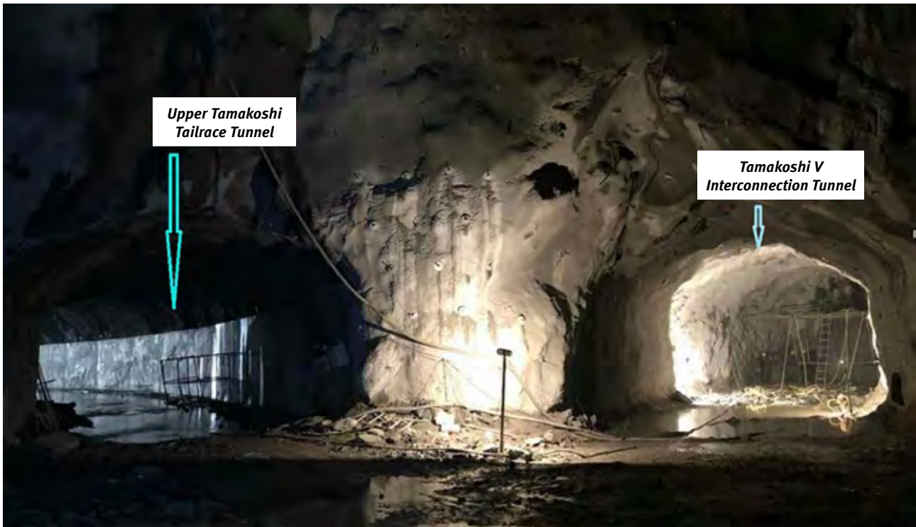
Interconnection System of Tamakoshi V Headrace Tunnel and Upper Tamakoshi Tailrace. (Source: https://tkjvc.com.np/ )
